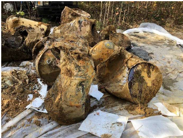
2 Crushed drums pulled from primary excavation pit
